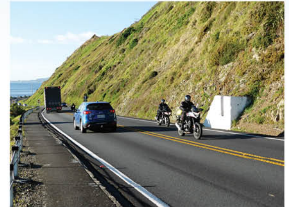
Second World War road block north of Pukerua Bay. Photo: Ashley Blair.
